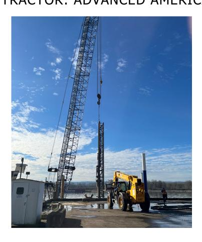
Diesel Hammer Installation of Wood Fender Pile
