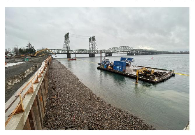
In Water Slope Grading Work Complete
