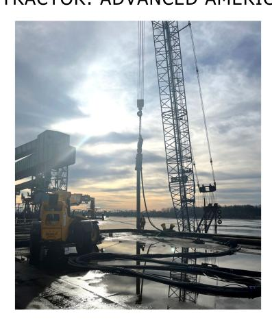
Vibratory Installation of a Wood Fender Pile
