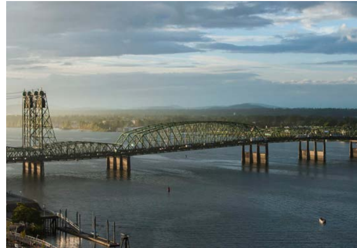
I-5 Columbia River Bridge
