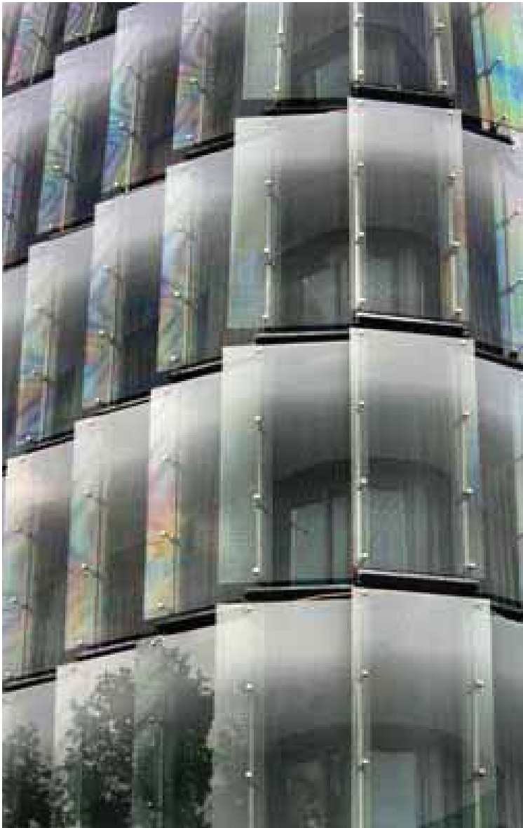
Galeo, part of a complex designed by Atelier Christian de Portzamparc in Issy les Moulineaux, France, has an external skin of printed glass scales which help to reduce reflections. Photo: Sipane
