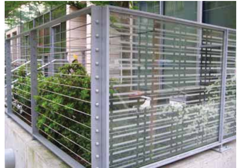
Visual markers on the balcony glass at the Eliot Tower provide some privacy and decrease strike hazards. Photo: Mary Coolidge
