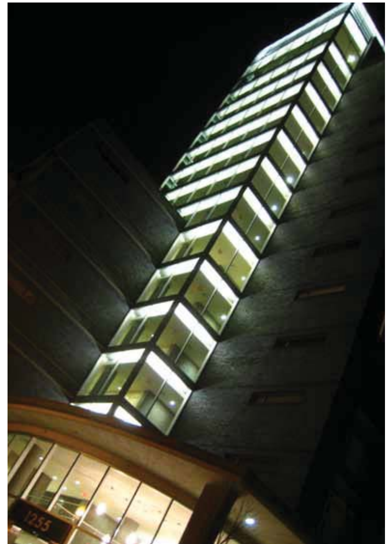
Light spill is apparent from this stairwell in the Pearl District, and could be minimized by exterior shielding. Photo: Mary Coolidge
