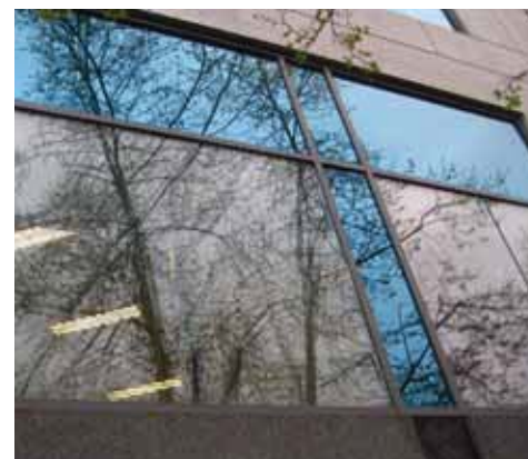
Tinted windows at the State Building readily reflect vegetation. More testing on colors and density is needed. Photo: Mary Coolidge
