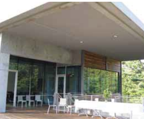
Overhangs block viewing of glass from some angles, but do not necessarily eliminate all reflections. Photo: Christine Sheppard, ABC
