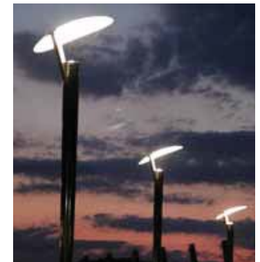
Cut-off shields can reduce lighting loss and permit use of lower wattage bulbs, resulting in lower costs. Shielded light fixtures are widely available in many different styles. Top photo: Susan Harder; bottom photo: Dariusz Zdziebkowski, ABC
