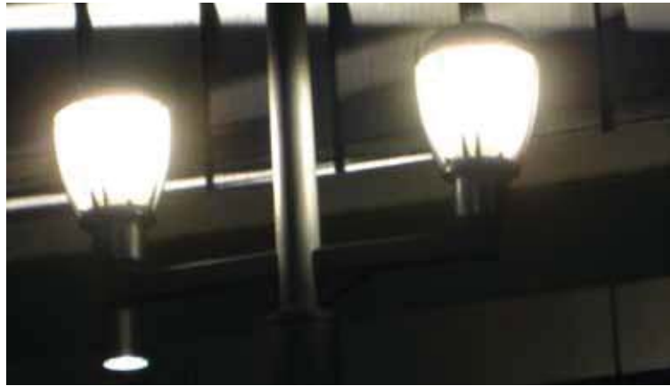
Though newer acorn-style light fixtures in South Waterfront have incorporated some shielding design, full cut-off improvements to the design of these fixtures would reduce contribution to light pollution. Photo: Mary Coolidge
