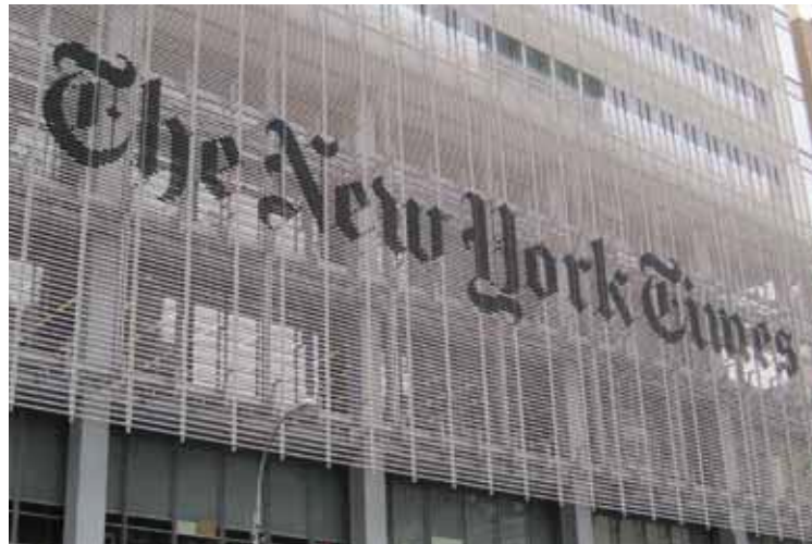
The façade of the New York Times building, by FX Fowle and Renzo Piano, is composed of ceramic rods, spaced to let occupants see out, while minimizing the extent of exposed glass. Photo: Christine Sheppard, ABC
