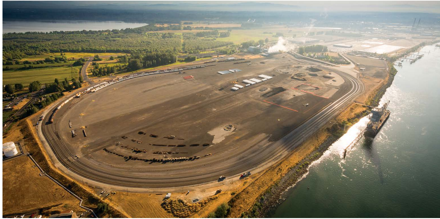
The Vancouver Energy project proposes to lease 42 acres at Terminals 4 and 5 for a crude oil transload facility
