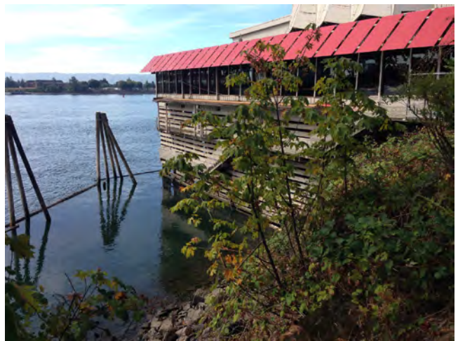
RIPARIAN CONDITIONS UPSTREAM OF PIER
