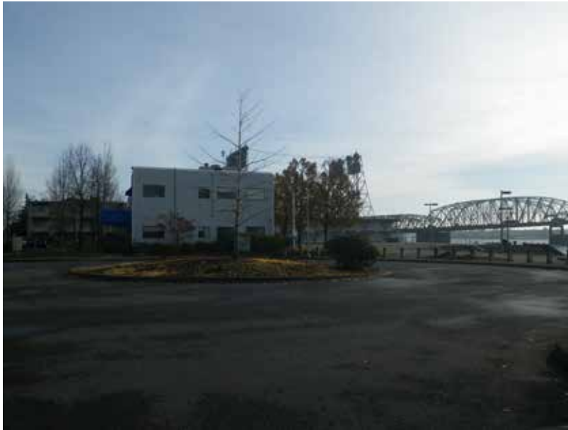
Photo 5. A traffic circle is located along the western boundary of the project area, next to the Columbia Shores building. The view is towards the southeast.
