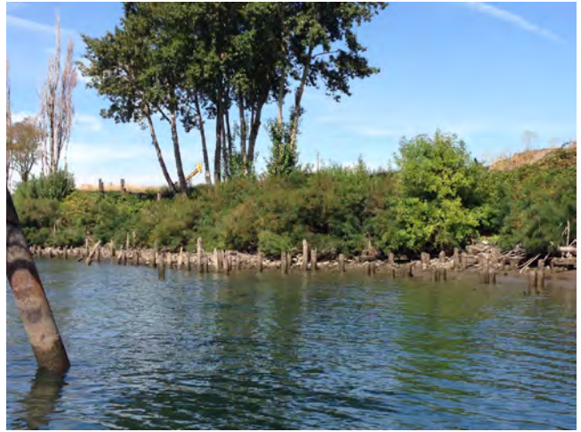
EXISTING TIMBER PILINGS DOWNSTREAM
