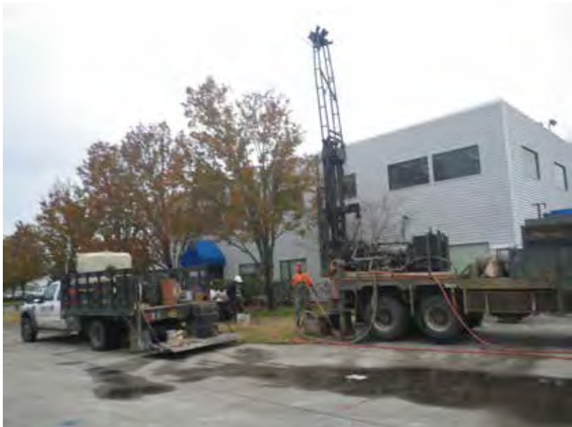
Photo 3. Overview of bore hole B2 excavated in front of the Columbia Shores building in the western portion of the project area. The view is towards the northwest.
