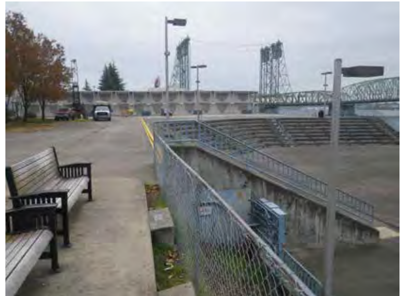
Photo 4. Overview of the project area showing public areas and the outdoor amphitheater. The Red Lion Hotel and Interstate Bridge are in the background, and bore hole B2 is on the left side of the photo. The view is towards the east.
