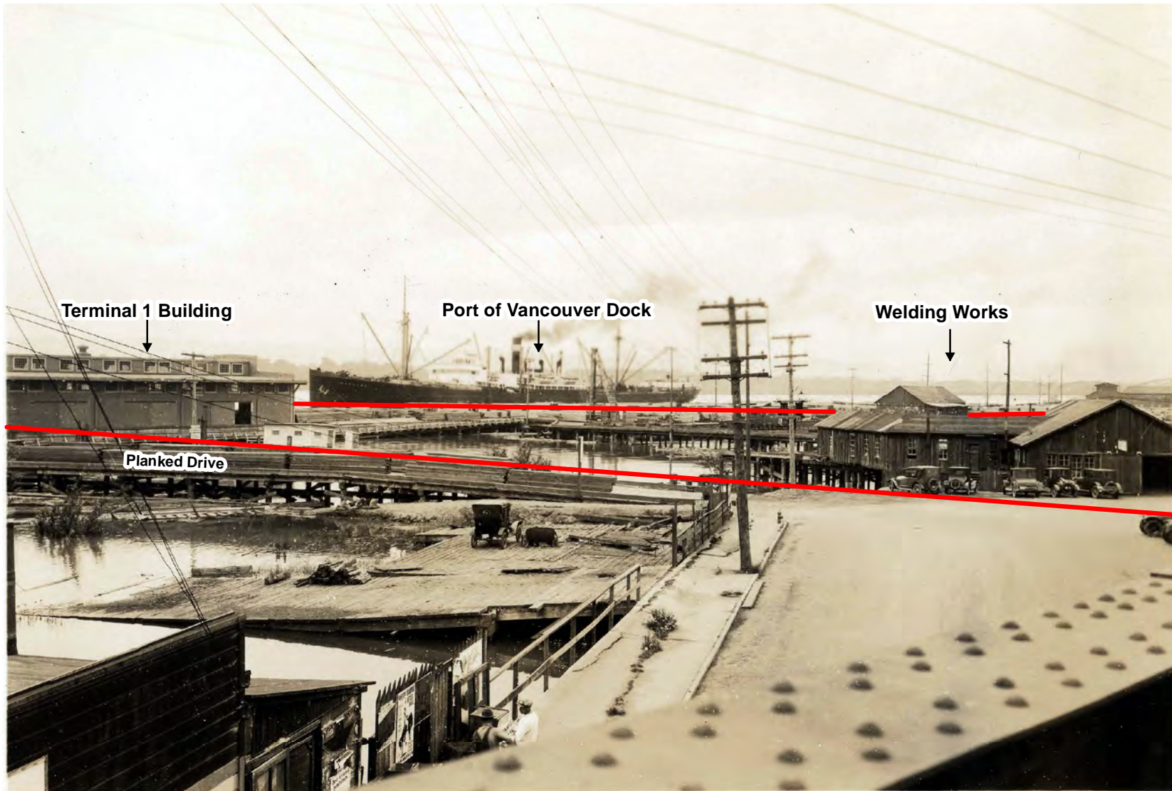
Figure 7. Overview of project area circa 1930. The view is towards the southwest from the BNSF railway overpass over Washington Street. The red line marks the approximate boundary of the current project area.
