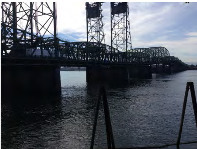
VIEW OF I-5 BRIDGE FROM HOTEL
