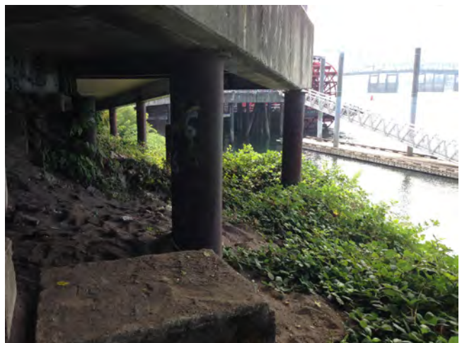
VIEW UNDER PIER DOWNSTREAM
