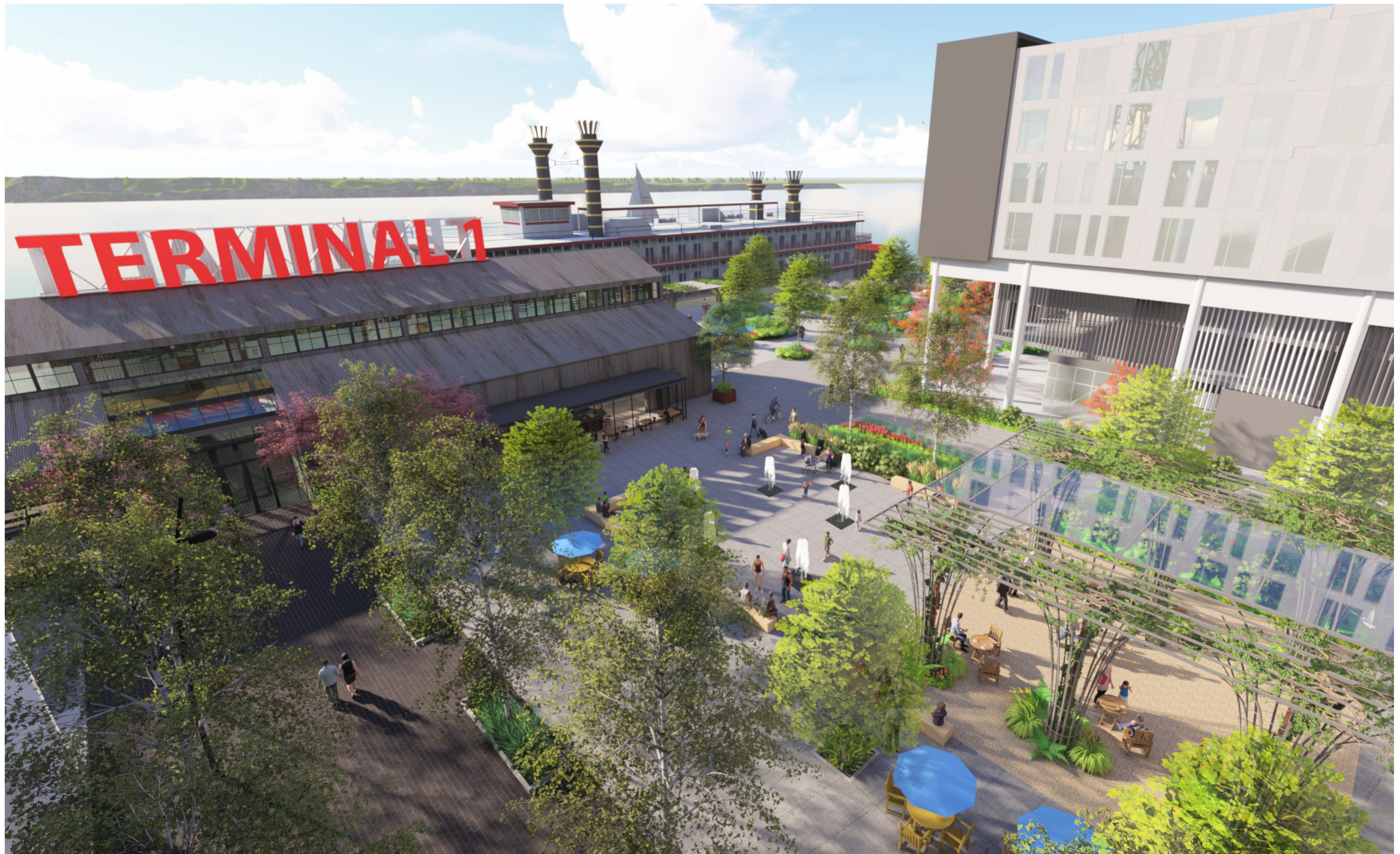
MARKET PLAZA FROM ADJACENT BUILDING LOOKING WEST
