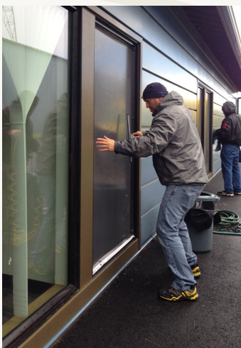
Left: Workers apply CollidEscape bird safe film on port building windows Top Right: Example of SOLYX SX-BSFV bird safe film used in industrial park Bottom Right: Example of SOLYX SX-BSFD bird safe film used in industrial park
